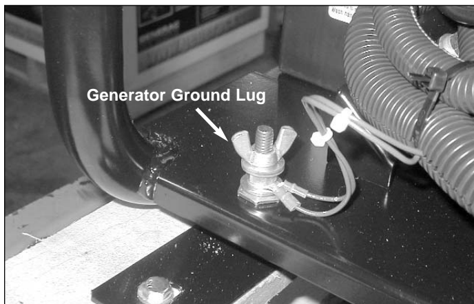
Figure 13 - Grounding the Generator
